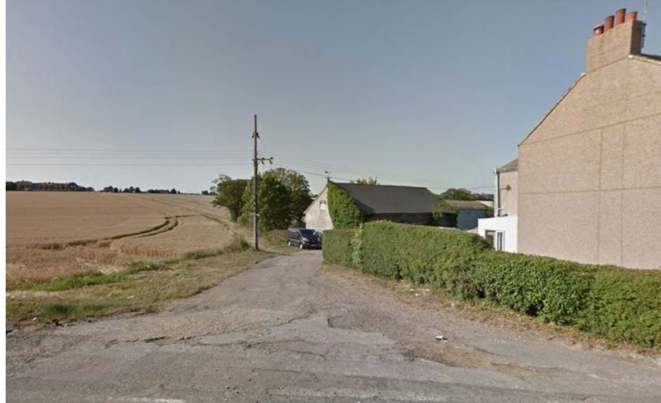
1 Public footpath accessed from Shottendane Road to the side of Twenties Cottages and agricultural buildings to the rear.
