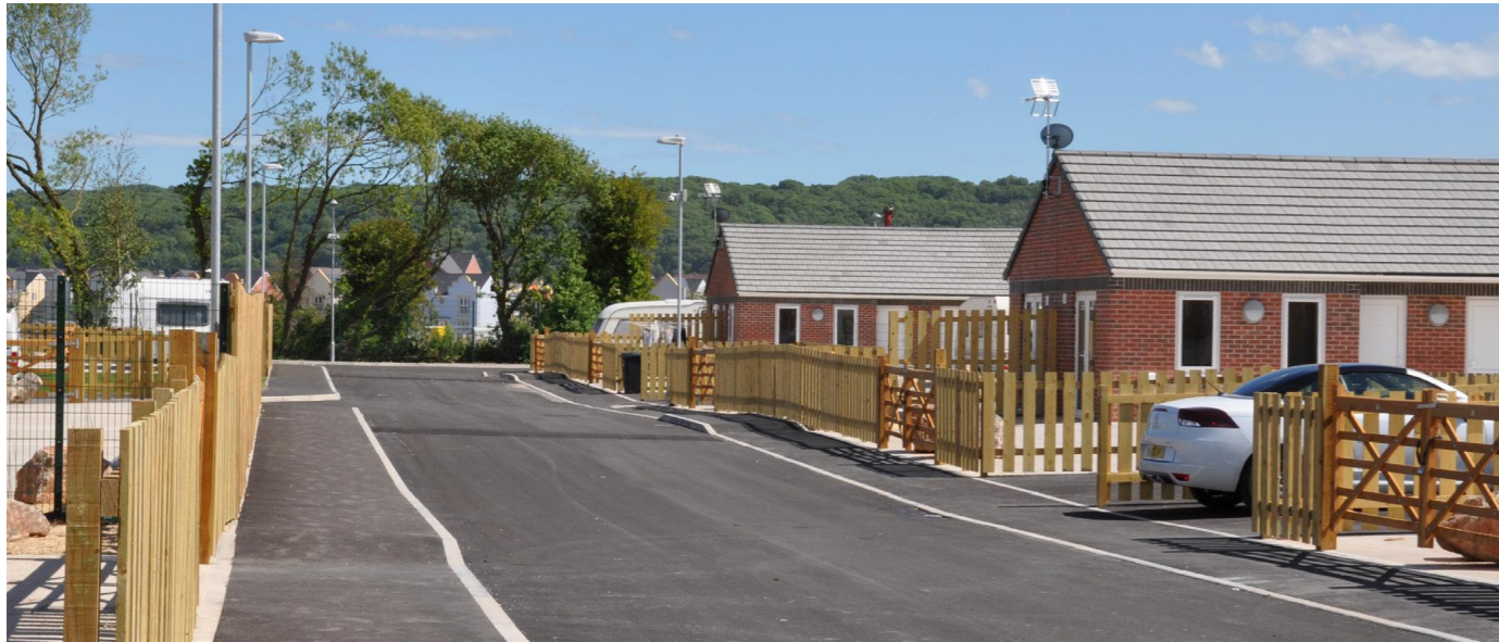
Elim Housing's Greenfields Way site
